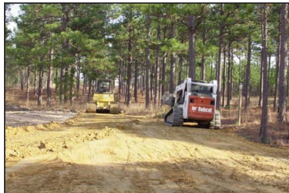
FIRELANE MAINTENANCE: HEAVY MACHINERY IS USED TO COMBAT EROSION ON FIRELANE THREE
