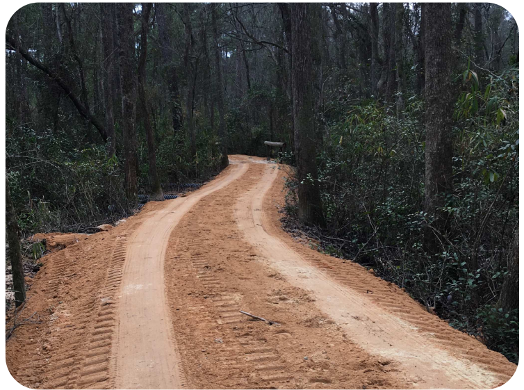
ADDITIONAL PIPES ADDED AT EDMISTEN CROSSING
