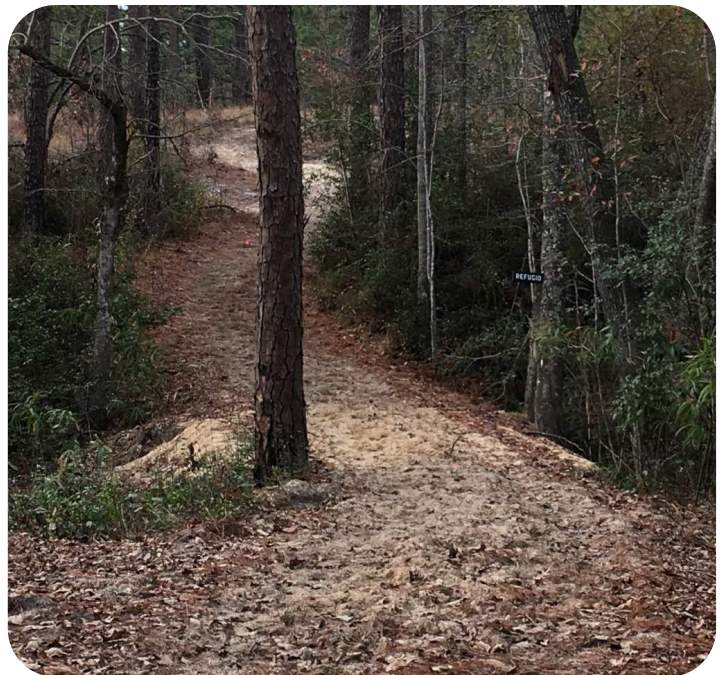
REFUGIO CROSSING, PIPE REPLACED AND CROSSING STABILIZED
