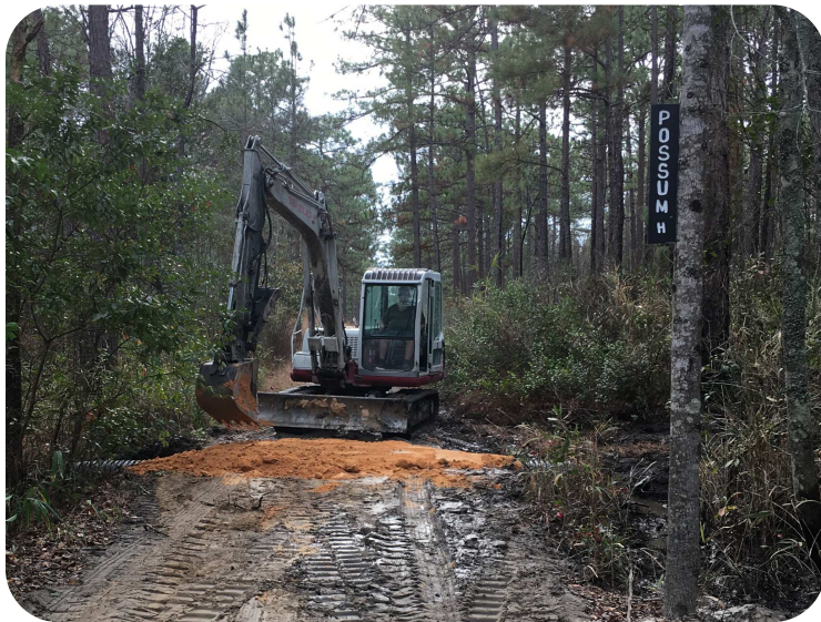
POSSUM HEAD CROSSING REPAIR BY KNOWLBROOK FARMS, INC.
