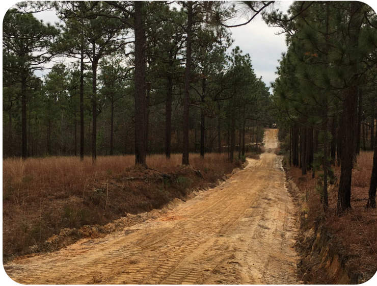
FIRELANE REPAIRS ON FIRELANE 1 EXT
